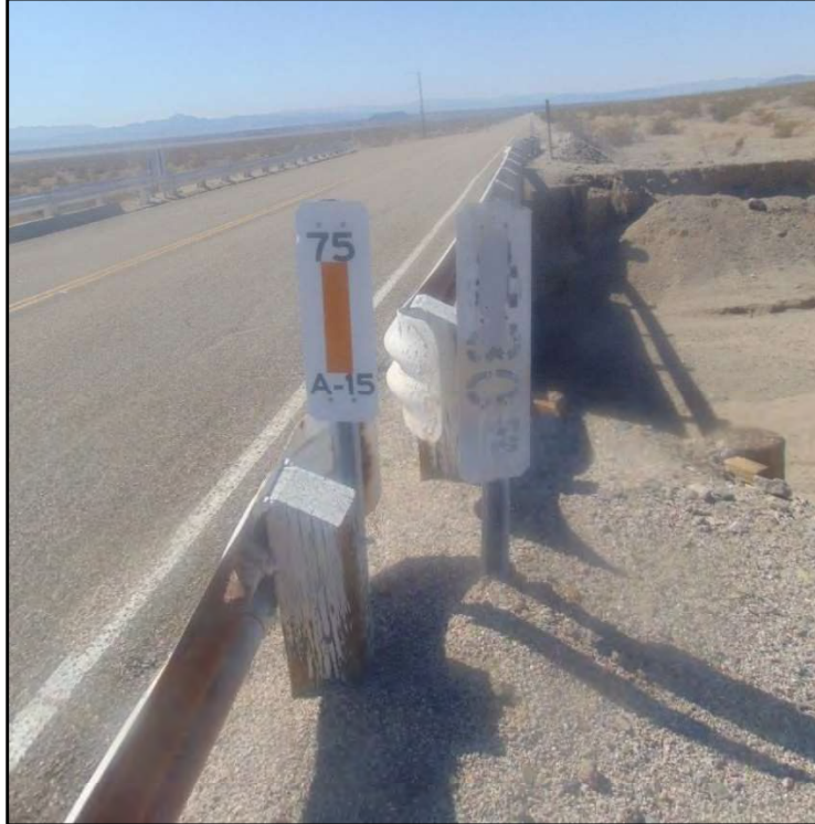
Photograph 1. Detail of two types of paddleboards. The one to the left is modern. The one to the right is an example of the late 1950s Paddleboard, subject to the protective measures in this SOIS Action Plan.
