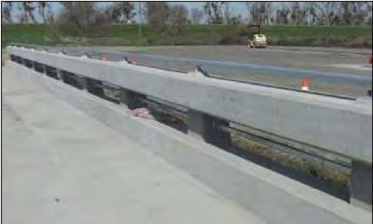
Completed Type 85 Barrier
