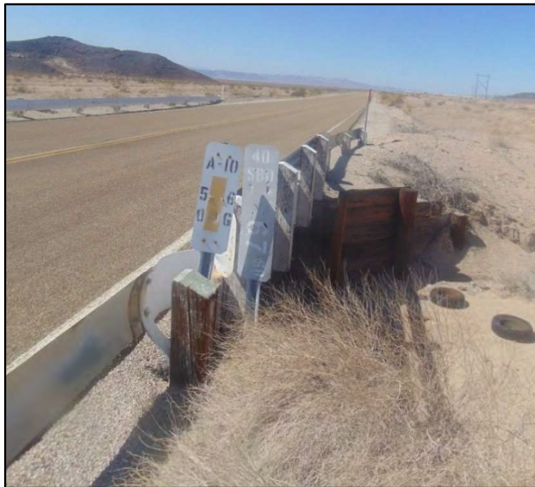
Photograph 2. Another example of paddleboards present at the bridge locations. The one to the left is modern. The one to the right is an example of the late 1950s Paddleboard, subject to the protective measures in this SOIS Action Plan.
