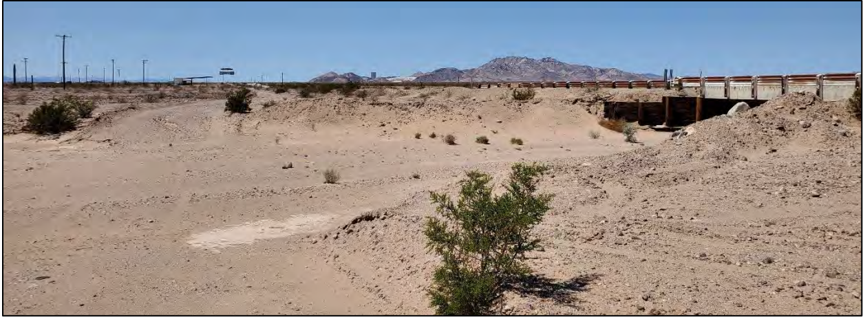
Figure 6. Lamego Ditch Bridge overview
