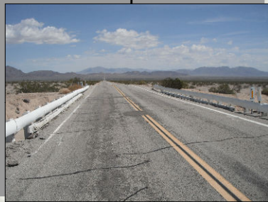
Photo 1 - Ground View of Bridge
