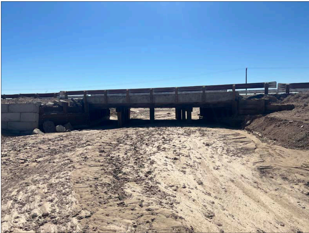
Photo 2. Overview of the Lamego Bridge (Bridge 85) along Route 66, National Trails Highway.
