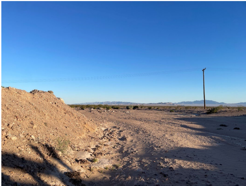
Representative Photo 2. Representative photo of main channel that is conveyed below the bridge. Photo of Lamego Ditch, facing south.
