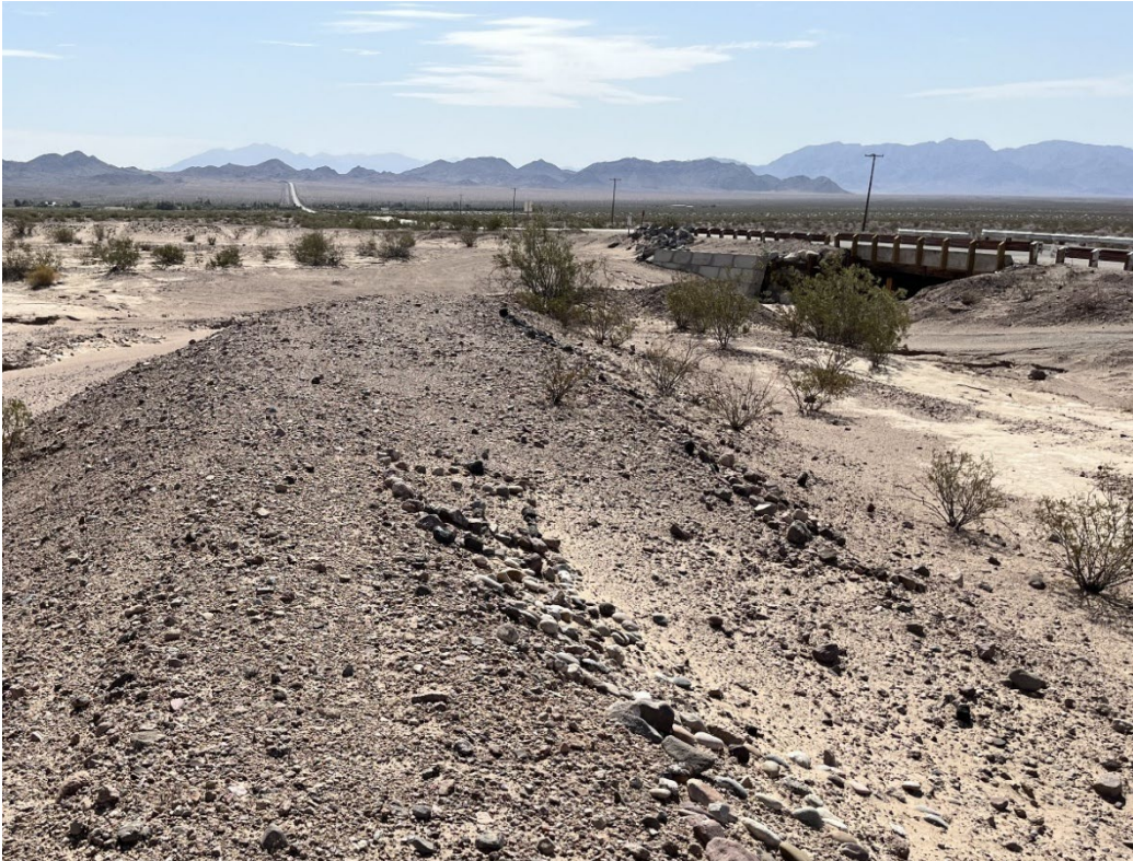
Representative Photo 6. View east from north of the NTH.
