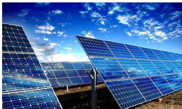
Figure 5: Solar Panels (source: http://www.thealternativedaily.com/solar-energy-bright-future/ )
