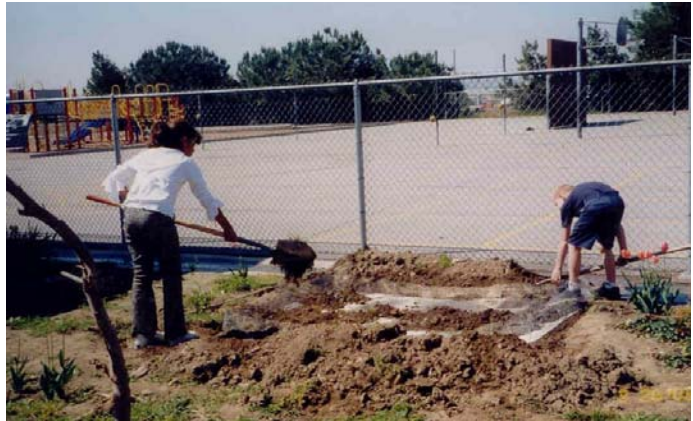
Filling in with dirt.
