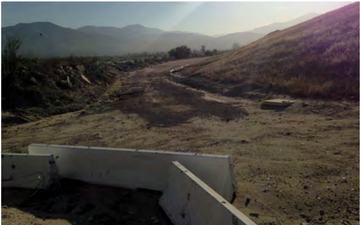
Photo 2. Access road alongside the landfill to the south. Looking east.
