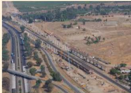
SAN JOAQUIN RIVER VIADUCT
